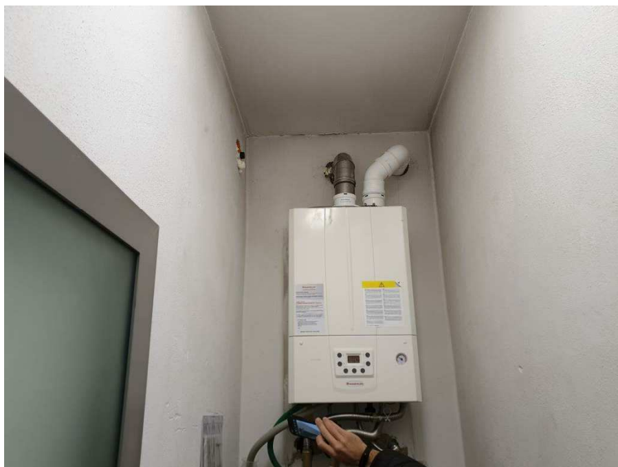
Vista 7 – Piano Terra
